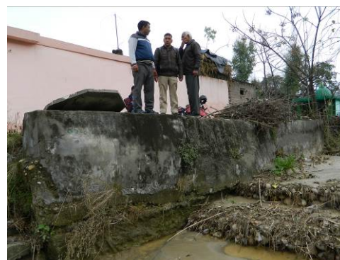
Eroded Concrete Embankment
