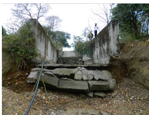
Partially Collapsed Water Channel (Dry Season)
