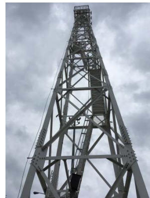
Photo 2: Navigation and support system (Additional Output)
