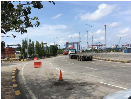
Photo 1: Improvement site of existing road inside the Port, which was developed by IPC II's Funds
