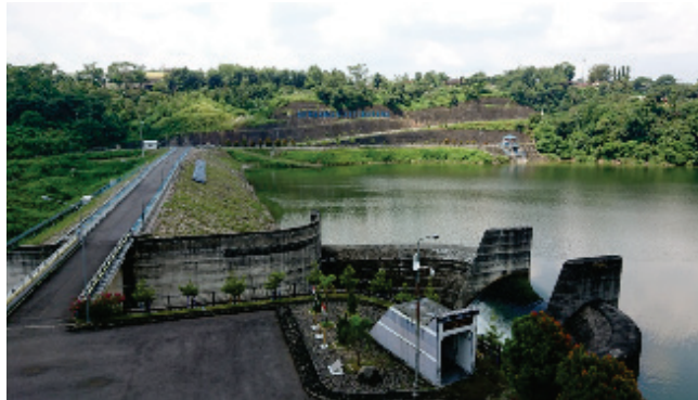
The Jatibarang Multipurpose Dam
