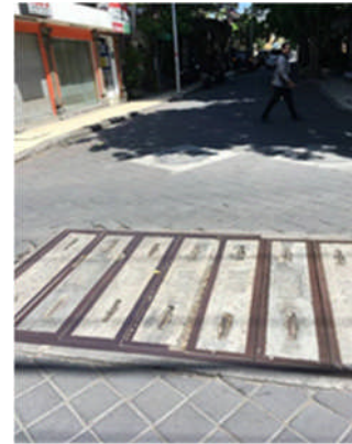
Manhole-type Pump Station Developed under this Project
