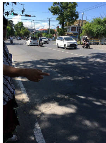
Photo 2: Developed Sewerage Area by This Project
