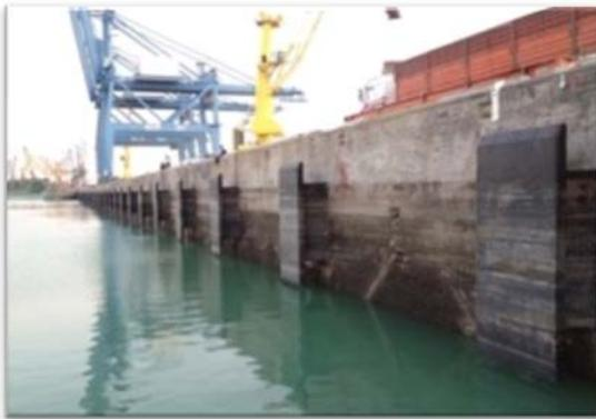
Photo 1: Fenders Installed by This Project<sup>12</sup>
