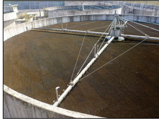
Trickling Filter
