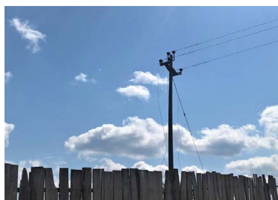
Theft damages of distribution facility (Loreto)
