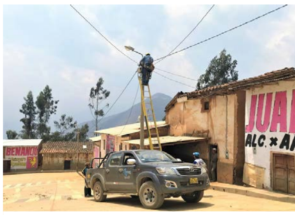
Maintenance of Street Lights (Huánuco Region)
