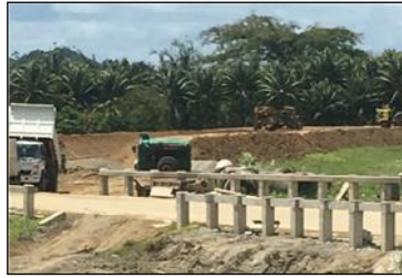
Main irrigation canal under construction in the Bulao Service Area
