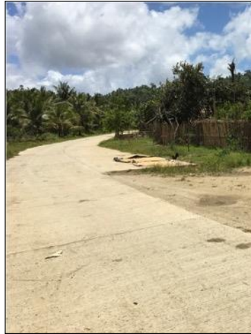
Farm-to-market road between Las Navas and Bulao (concrete paved and upgraded to a national road after this project)
