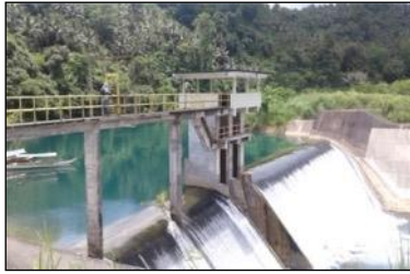
The completed Catubig Dam (Photograph provided by the executing agency)
