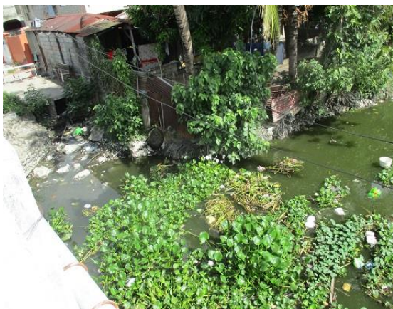
A local drainage channel adjoining the project site, necessary to remove silting accumulated on the riverbed and plants on the river surface
