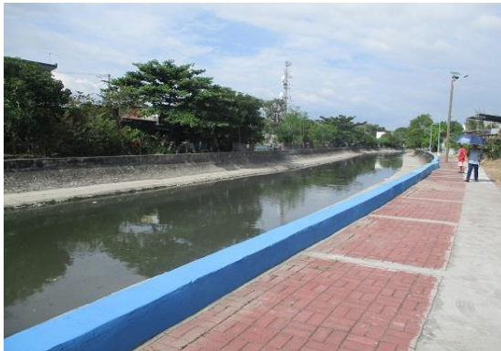
Dredged and widened local drainage channel
