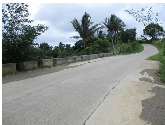
Paved farm-to-market roads in the sub-loan project. Tomato fields and sugar cane fields are scattered along the roads. (Province of Batangas)
