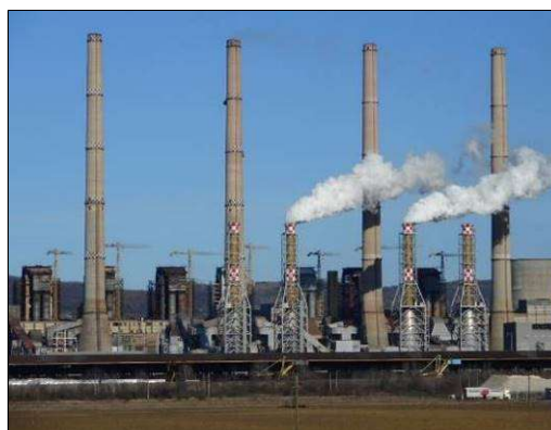
FGD including four absorber towers in the front
