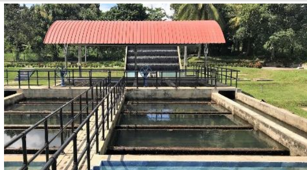
Mahaoya Purification Plant (newly constructed)
