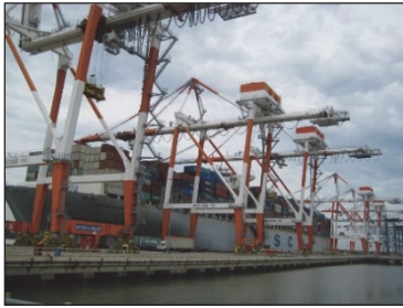
Berth and Container Cranes
