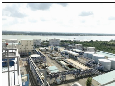
Photo 1: O Mon Power Station Fuel Tanks
