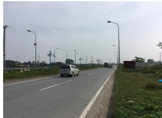
Road Developed under the Project
