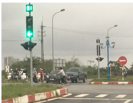
Picture 1: Traffic Light Installed on Road
