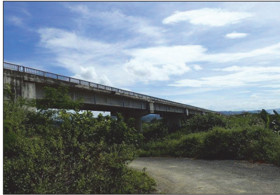
Dak Pri bridge (Dak Nong province) rebuilt by this Project
