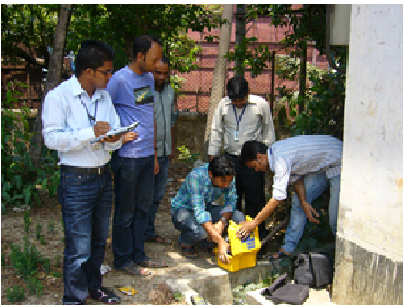
Leak detection using a mobile ultrasonic flow meter
