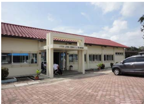
Exterior of Dumai VTS Center Building
