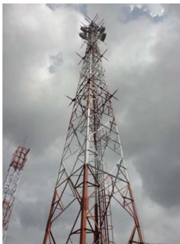
Radar Scanners and Multiple Transmission Parabolic Antennas at Dumai VTS Center
