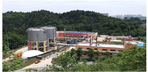
Food waste disposal center at Xining City. The facility was established by China and is being operated since 2016. It is currently operating by applying the lessons learned through the project.
