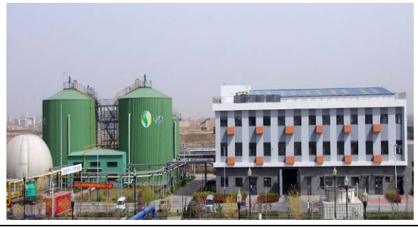
Food waste disposal center at Qingdao City. The facility was established by China and is being operated since 2013. It is currently operating by applying the lessons learned through the project.
