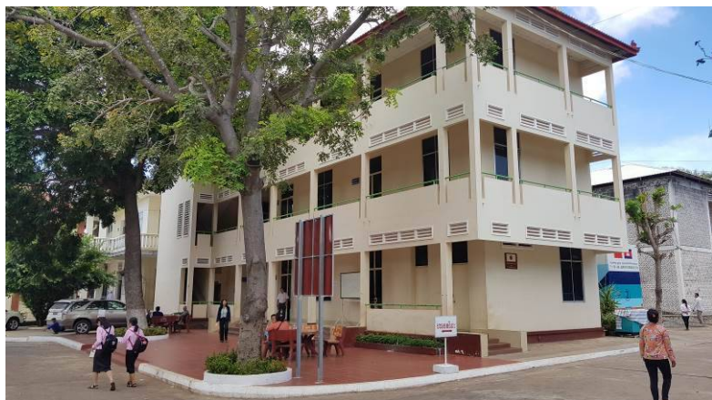
Exterior Structure Training Unit of Kampong Cham Provincial Hospital
