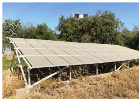
Rehabilitated rural water supply using solar system (Water Supply)
