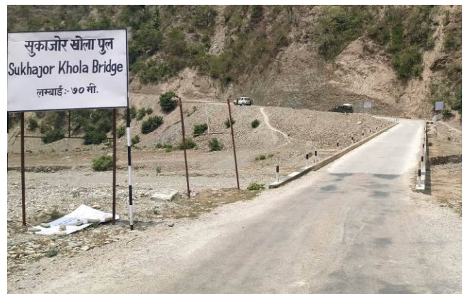
Sukhajor Khola Bridge (Ramechhap) linking Manthali, Ramechhap and the western part of Okhaldhunga district
