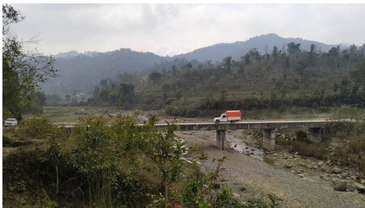
Dhamile Khola Bridge (Sindhuli) linking Sindhulimadi and the rural areas
