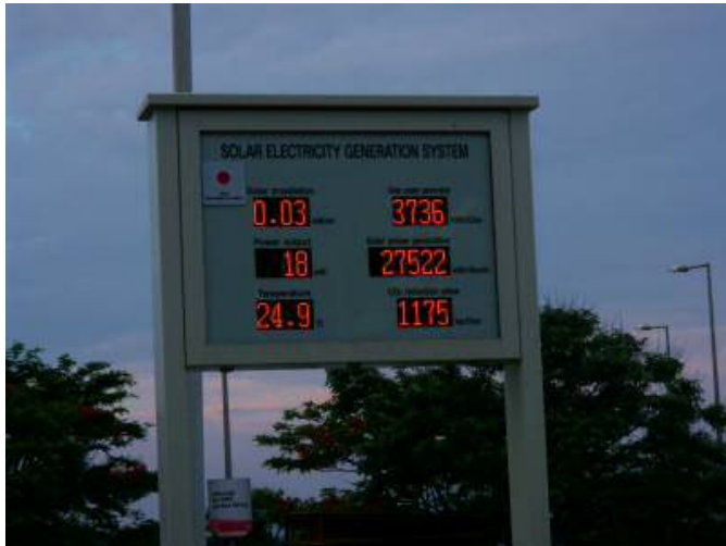
Display board indicating the energy amount being generated by the facility
