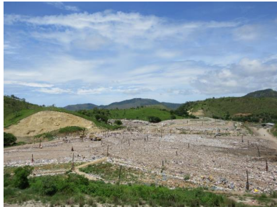
Baruni Landfill, improved through this project (Papua New Guinea)
