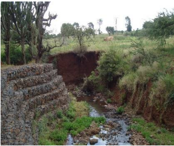
Riverbank protection gabions constructed during the project in Isiolo Sub-catchment.
