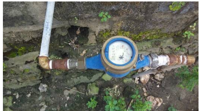
The water meter connected to single household; old style used by the phase 1 project (At Makadara area)
