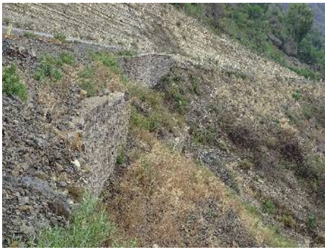
Retaining wall constructed by Ethiopian Roads Authority
