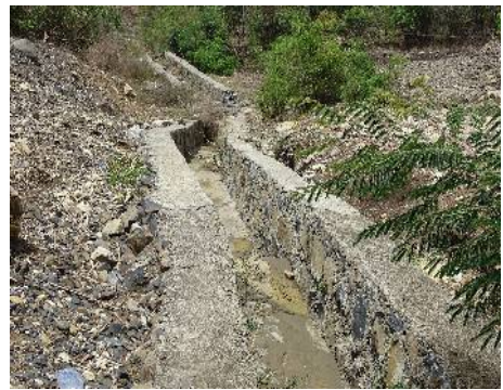
Ditch constructed by Ethiopian Roads Authority
