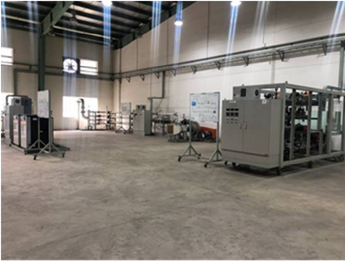
The Energy Management Training Center in HCMC
