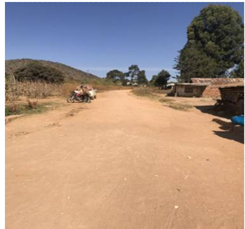
Wenda -Mgama road in Iringa Region one of the pilot projects of the project
