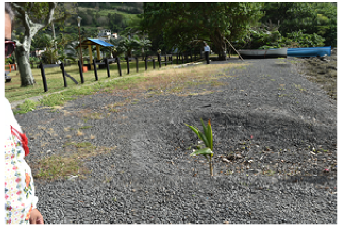
Flexible revetment along the coast of Grand Sable keeping a space for fishing activities for fishers
