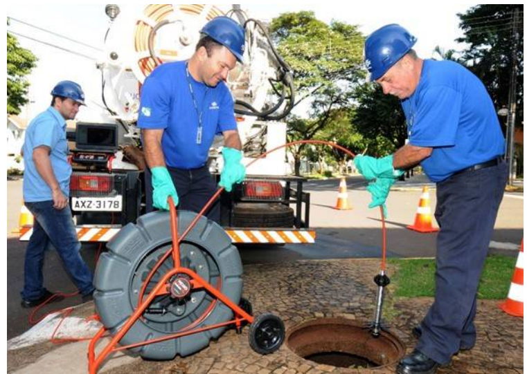
Diagnosis of Sewerage Pipe Network
