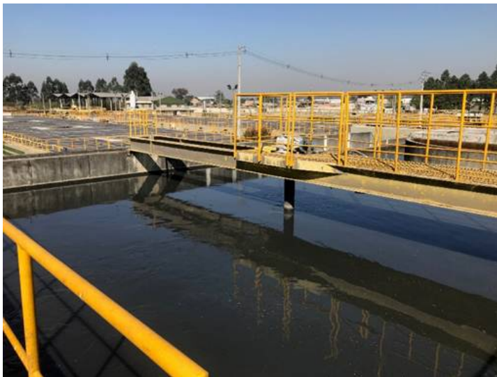
Sewerage Treatment Plant in Atuba Sul
