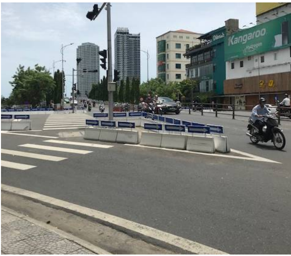
Le Duan- Tran Phu intersection: one of improved intersections on Le Duan Corridor
