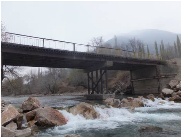
Bridge (Myrzake-Kara-Shoro) before repair.
