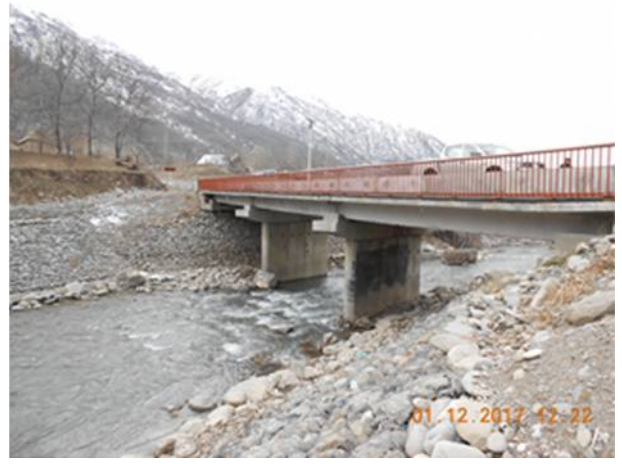
Bridge (Myrzake-Kara-Shoro) repaired in 2016.
