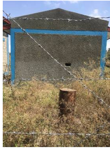
The test borehole developed in this project and an operation building constructed by USAID (behind) which are to be utilized for water supply to a nearby town
