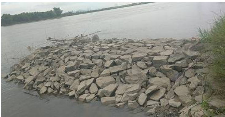
Small-scale River Bank Protection Work in Ha Tinh Province
