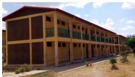
Secondary school constructed by this project
