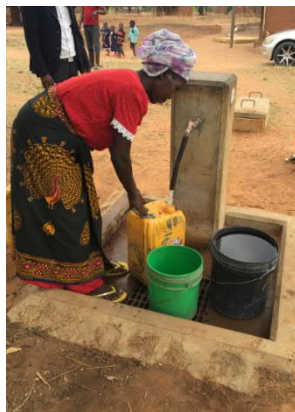
Level 2 water supply facility (Tabora municipality)
