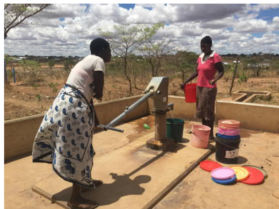
Level 1 water supply facility (Sikonge district)
