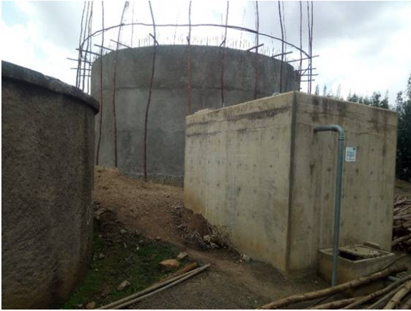
Water reservoirs (left: existing, right: newly constructed in this project, behind: newly constructed by TWU for the use by an additional community)
