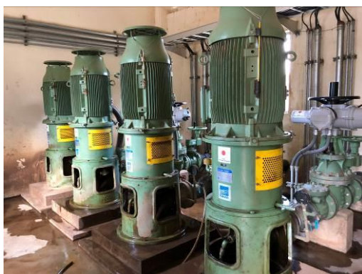
Pumps at the newly constructed intake facilities
