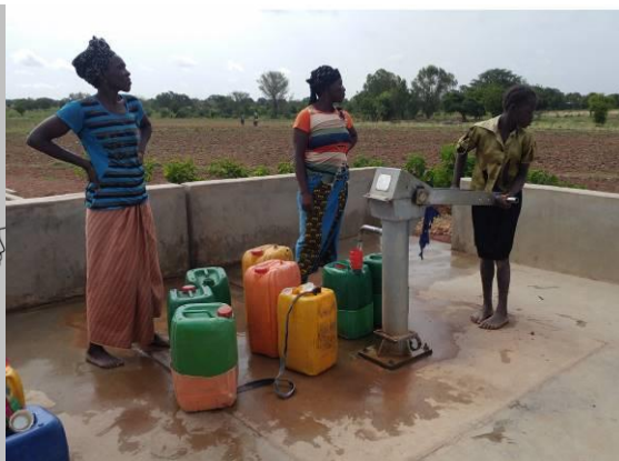
PMH constructed by the project
