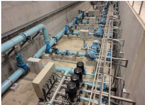
Transmission Pump and Distribution Pump (Battambang)
