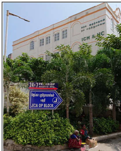
Outpatient building constructed by the project
