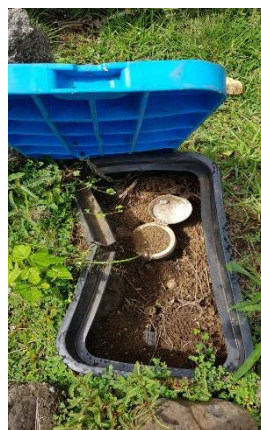
Water Supply Equipment (Water meter)
