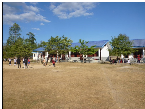
School buildings constructed by this project
