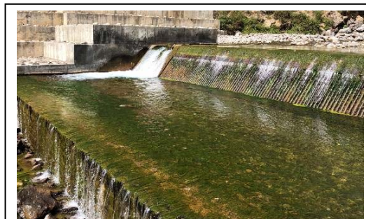
Intake of Syarpudaha Micro-Hydropower Station
