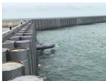
Photo: Pond-type water intake
