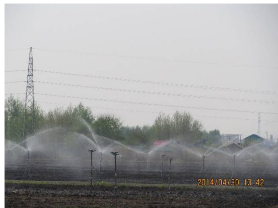
Sprinkler system introduced under the Project
