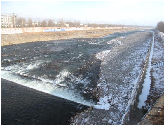
Revetment protection work under the Project
