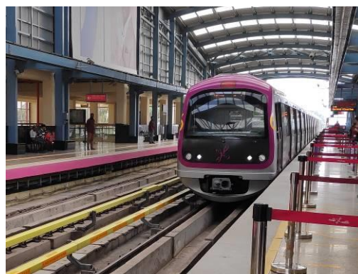
East-West line of Bangalore Metro constructed by the project
