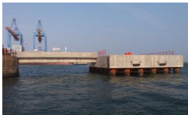
Mooring dolphin constructed by this project
